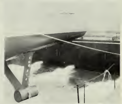
(10) Drydock flooded down for launching
